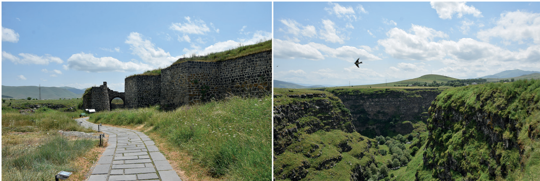
Fig. 2. Lori berd, castle. Entrance on the left and view from the Castle to the valley on the right. Photo taken by the author in 2022.
