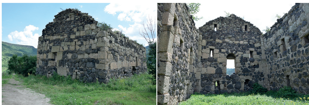
Fig. 8. Building within the territory of Hnevank 4 . Outside and inside photographed by the author. 2022.
